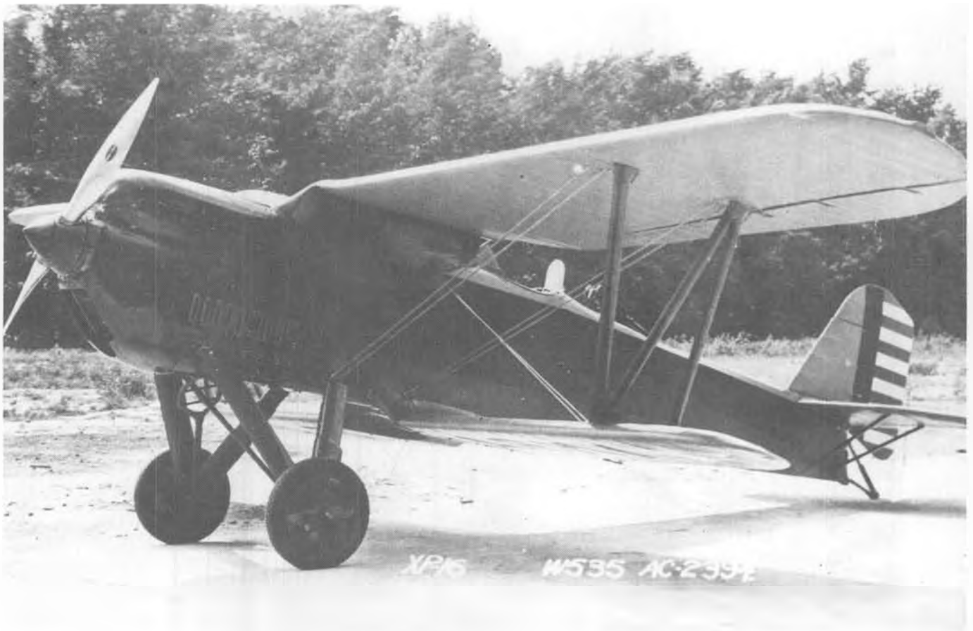
The one-only XP-16 was completed October, 1930. Supercharged Curtiss Conqueror of 600 hp gave the two-seater a top of 183 mph at 10,000 ft.
