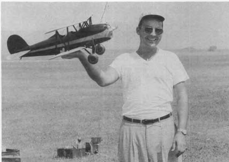
DOWN MEMORY LANE . . . RCMB's editor at Indiantown Gap Labor Day Weekend R/C Get-together, near Harrisburg, Pa., probably 1958. The Great Lakes was McCoy .09 powered (?), with Kraft single, Bonner Vari-Comp, rudder only. Stable flier. RCMB plan 9781.
