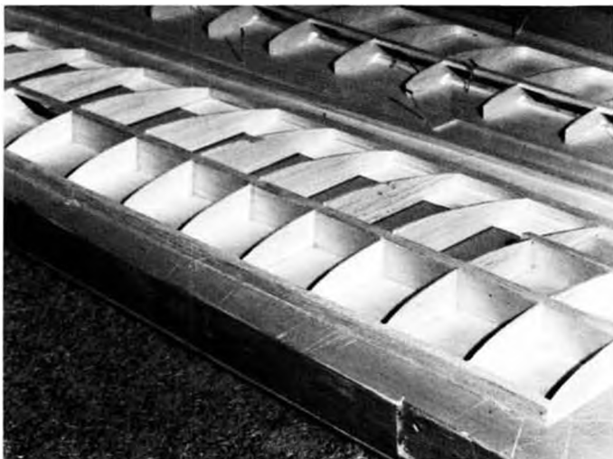
Structural design of wing allows almost complete assembly on bench before removal. Note those very important webs. Don't leave 'em out!
