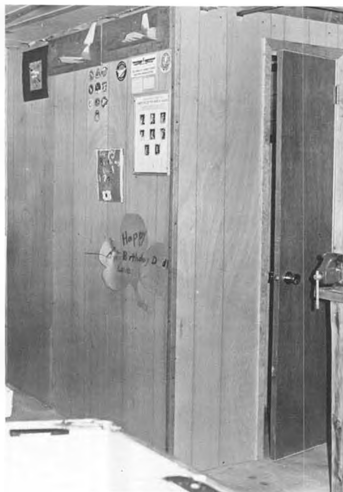
For home processing of black and white prints, Bob built this dark-room in a basement corner. Inexpensive panelling on 2x3's did it.
