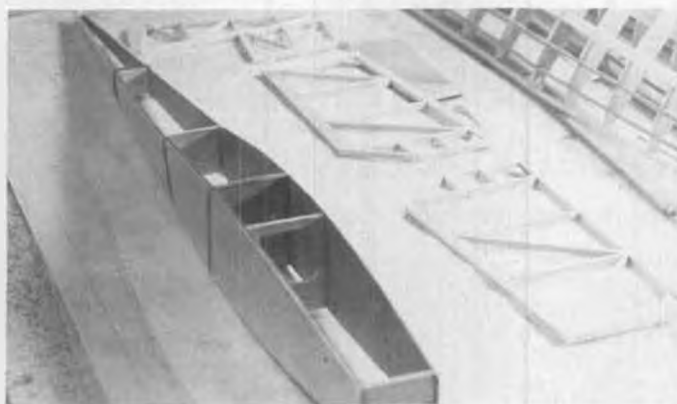
Fuselage structure without top and bottom sheeting. With full-length 1/64 ply side doublers, that fuselage should never break!
