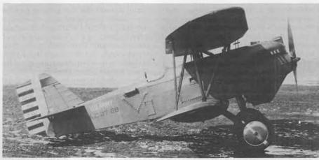
More changes on the McCook P-1B. Disc wheels with brakes were developed and the tailskid has been faired with wood. Fire extinguisher was still standard equipment . . . presumably for mechanics to put out ground fires. Pilot sure can't get to it in the air!
