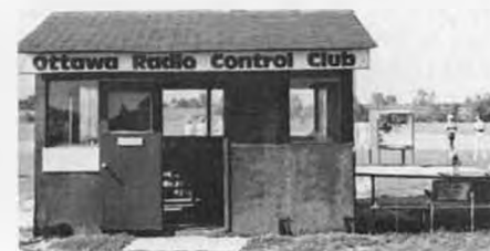
4. In the summertime, the SAM 86 clubhouse is used extensively. It's insulated for winter-time use too.
