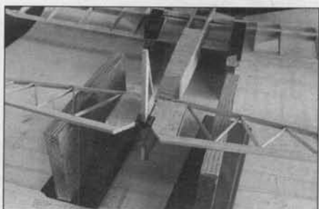
Stabilator alignment. Wing and stabilator on equal height blocks. Once in position, glue bearing blocks.
