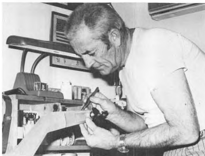
John is threading the tail rotor drive shaft into the coupling, with the aid of a pair of tweezers.
