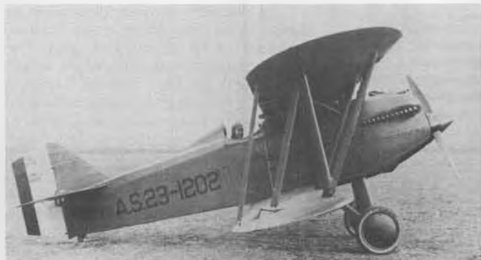
Radiator on PW-8 was hundreds of small brass tubes laid chordwise on top wing. Faster but far less maneuverable than PW-9.
