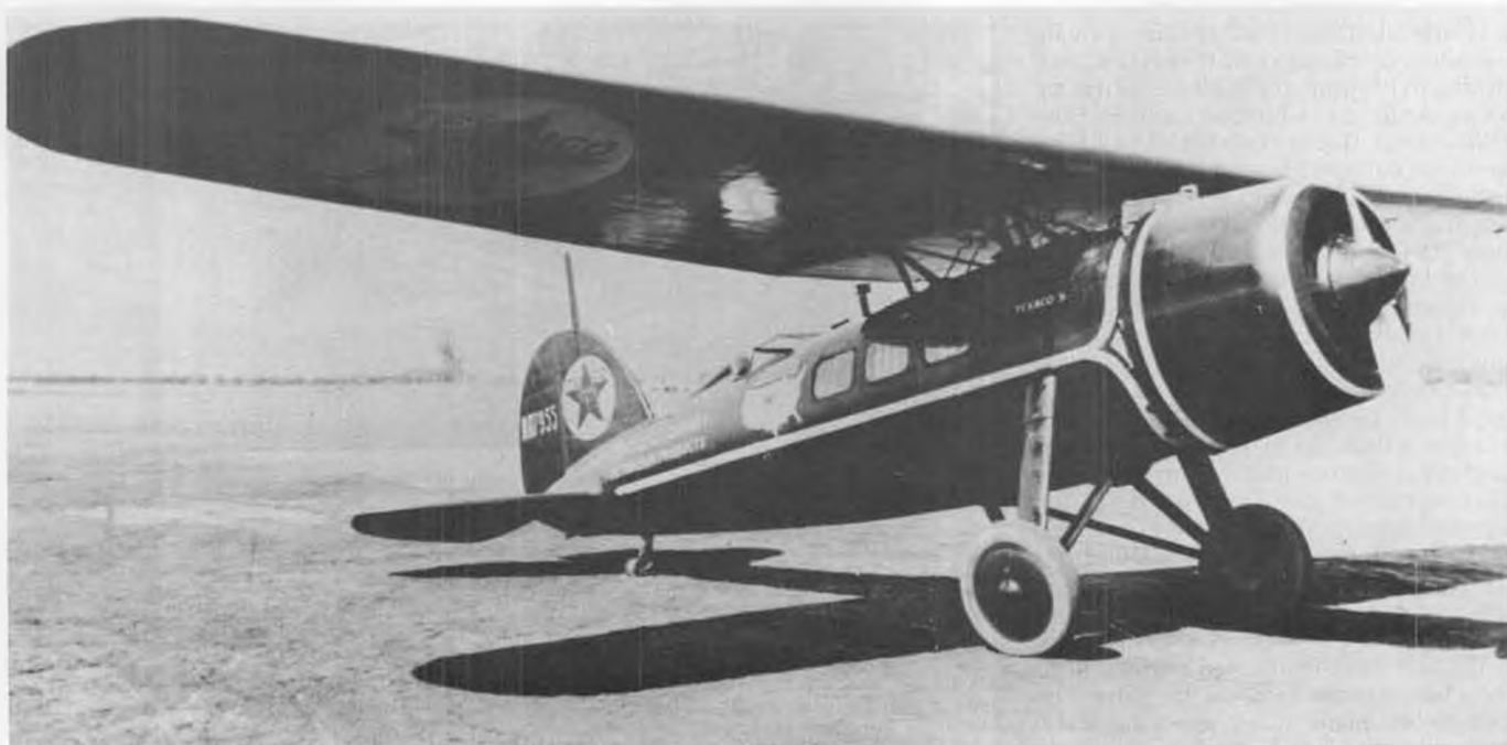
Capt. Frank Hawks flew his Lockheed Air Express "Texaco 5" for the Texas Company. Notice exposed oil cooler above cowling. The Air Express was Lockheed's third design.
