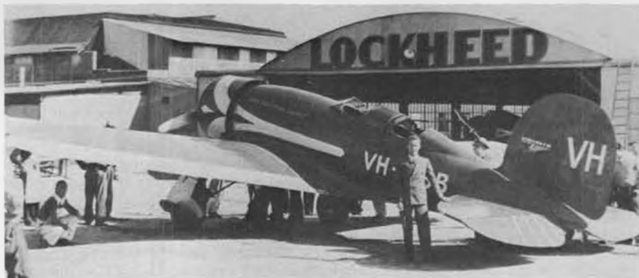
Sir Charles Kingsford-Smith stands by his Lockheed Altair, the fifth design, and first Lockheed to feature retract gear. He established several Pacific Ocean records in this plane.
