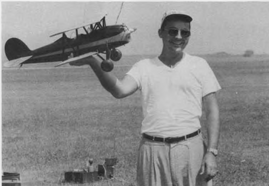
The writer with his first published model, about third R/C, one-inch scale Great Lakes Trainer with rudder-only control. McCoy .09 engine. For about 50 percent of every flight, no radio was used. It flew big, lazy circles to left. Radio mostly used to guide it back to landing area. Photo taken at Indiantown Gap, PA, 1957 or 1958.
