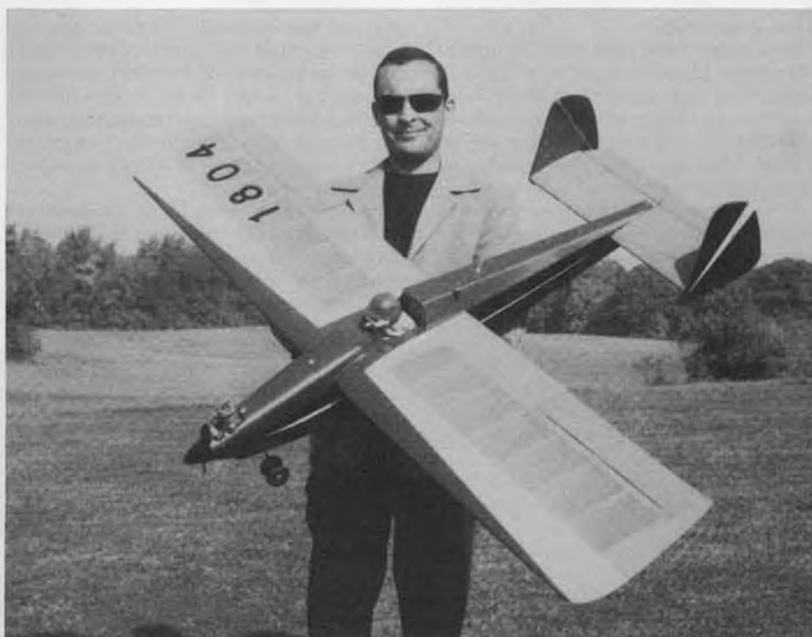
The writer and his "Torrero," designed by Willy Smith and published in an early RCM, around 1964-65. Engine was a Clarence Lee .45. Note also twin wheeled nose gear. Basically a Stormer, the thick wing, with full-depth, notched 1/8 spars, was strong and light. A real good flyer. Our first multi-proportional, using Don Brown's first, grey-box Quadruplex. Tired of seeing my photos? Come on guys, send in pics!
