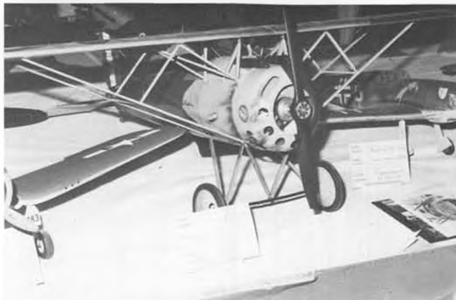
Morane Saulnier A-1 by Ed Spinks, Schenectady, N. Y., built to one fourth scale. Prop is belt-driven by offset mounted engine. It flies!
