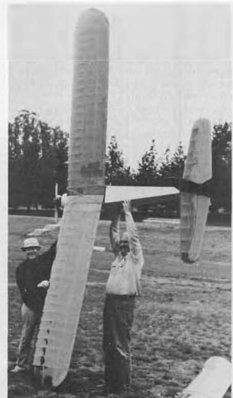
Fifteen feet of Dallaire Sportster! Builder Karl Tulp (left) and Ron Kiel share the load. Ron is also building a similar ship. Model has 4008 sq. in. of wing! Plans are available.
