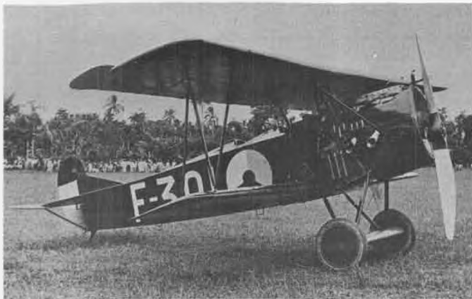
The Dutch East Indies Air Force flew D-VII's in the early '20's. Powerplant is a British Siddeley Puma engine.
