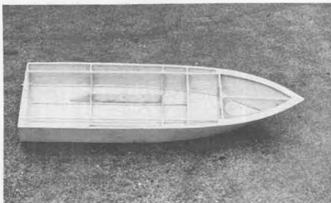
Engine bearers and deck stringers in place, ready for plywood deck sheeting.
