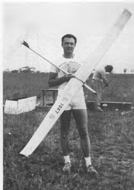
Two photos of Merv Buckmaster and his "Eldia 2 DC" original design A/2 Nordic. Elliptical tip dihedral is quite rare on F/F designs, but is sometimes seen on R/C sailplanes.
