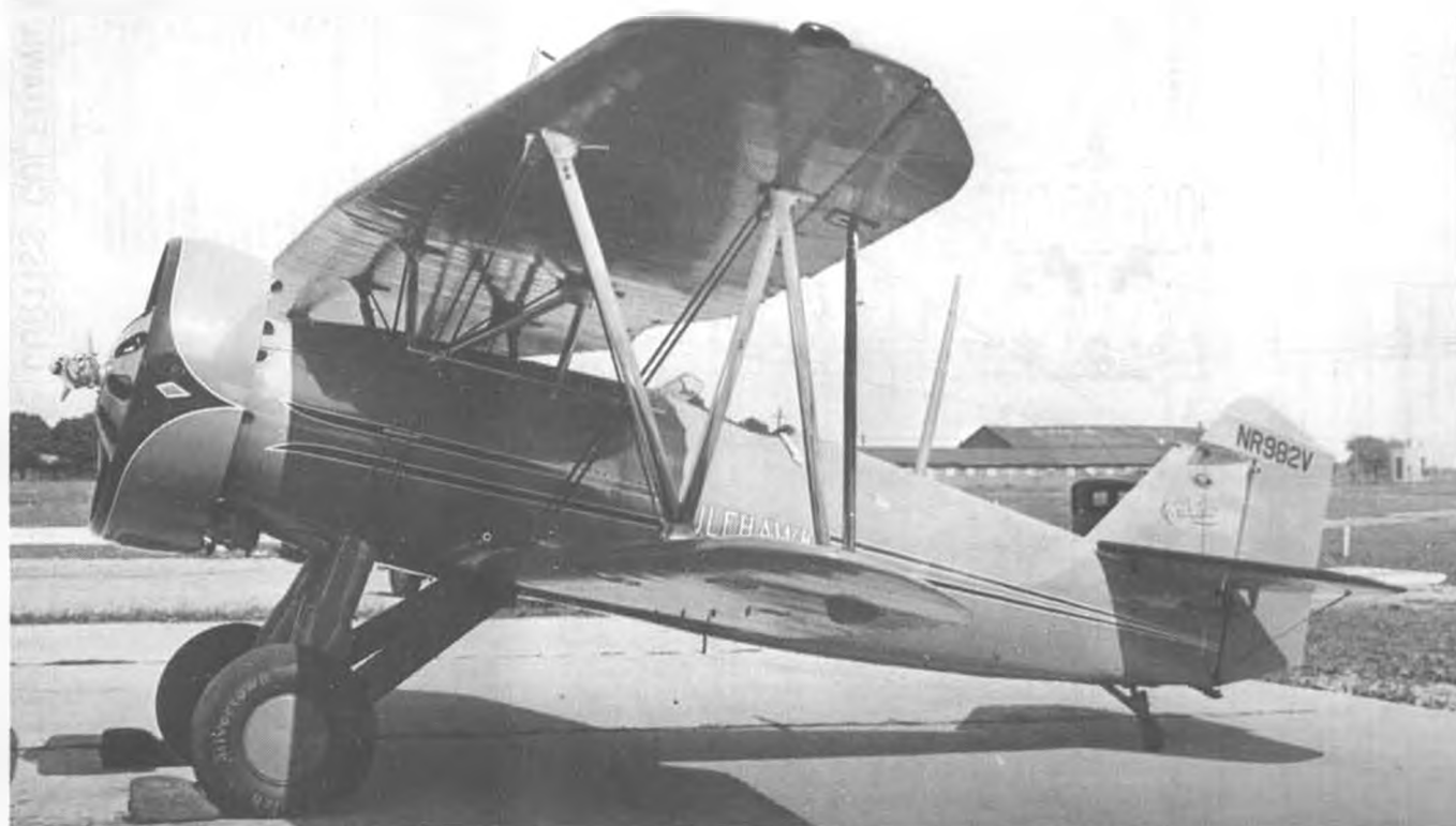
Al Williams' personal aerobatic plane, built by Curtiss, and following a crackup, was rebuilt at the expense of Gulf Oil Company, who thenceforth took over sponsorship and named it 'Gulfhawk.' Rebuilt ship had aluminum covered fuselage and fin, low pressure tires, Wright Cyclone engine.
