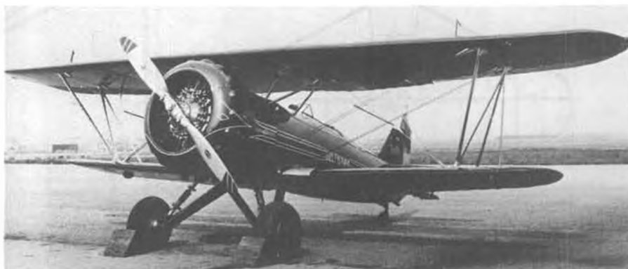
Later revision of Gulfhawk IA included a smaller diameter drag ring with blisters to clear the valve covers and deeper overall chord. Note uncovered shock struts.
