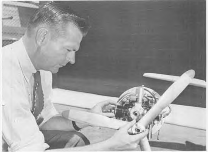
Ernest G. Stout, manager of Advanced Transportation Systems at Vultee, fitting special three-bladed prop on Ohlsson engine.
