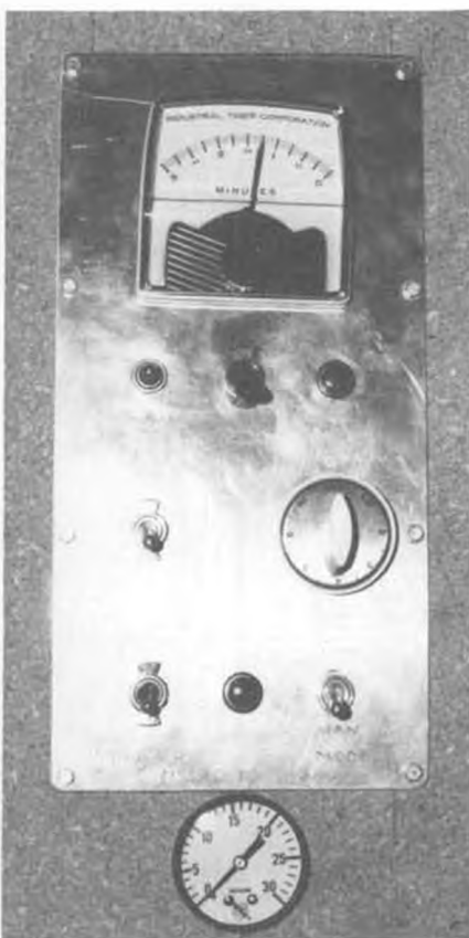
Close-up of control panel, with timer and heat controls. Plans available.
