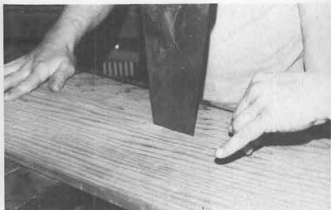
Final inch on either side of break point is cut with hand saw.
