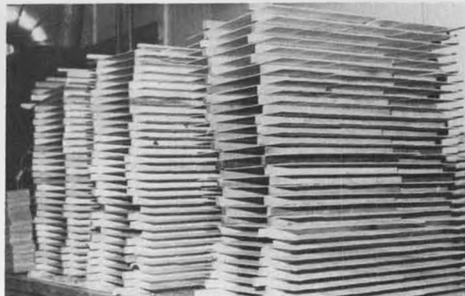
Wood is dampened before die-cutting, which prevents "die-smashing". Then it is stacked between spacers for room temperature drying.
