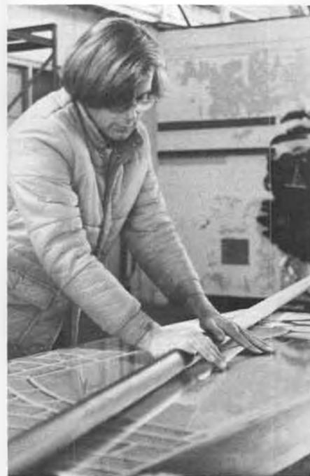
Well-known modeler Bill Watson is seen here rolling a structural tube of carbon fiber for the Gossamer Albatross.
