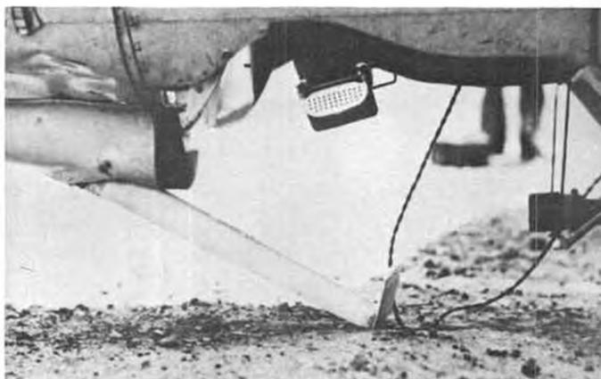
Landing on the Hampton Roads carrier landing platform: "... the left tire (of the XF11C-2) blew out; the left wing struck the deck and the plane nosed over and skidded on its back for a distance of about 20 feet." Photo from the Nat'l Archives.
