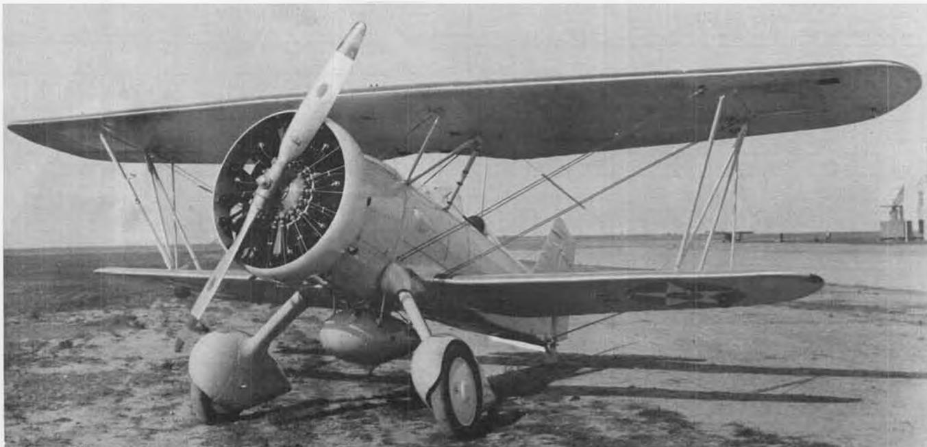
The first of many changes. This F11C-2 has high-pressure tires, teardrop auxiliary fuel tank, and the pivot point for the bomb cradle has been moved forward. Note that the Navy censor has deleted the arresting gear hook. Photo courtesy of Smithsonian NASM.
