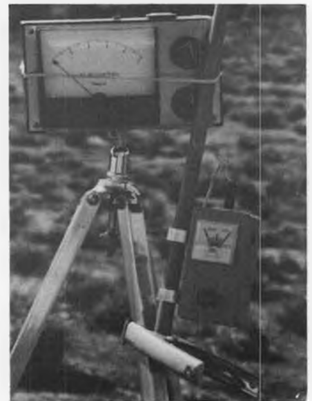
Tom Cashman's thermal detection system; temperature sensing unit from device for detecting warm air leaks in home insulation!
