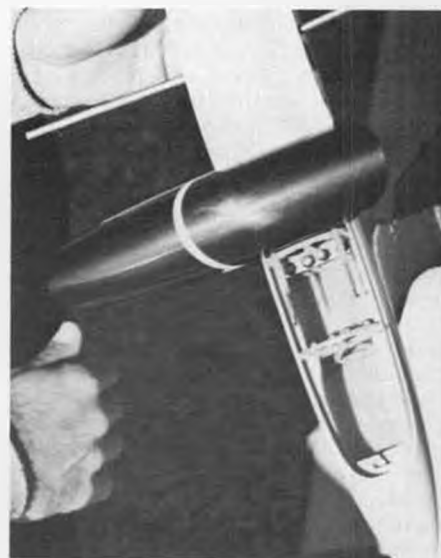
Radio compartment of Maria. Note lightened bulkheads.
