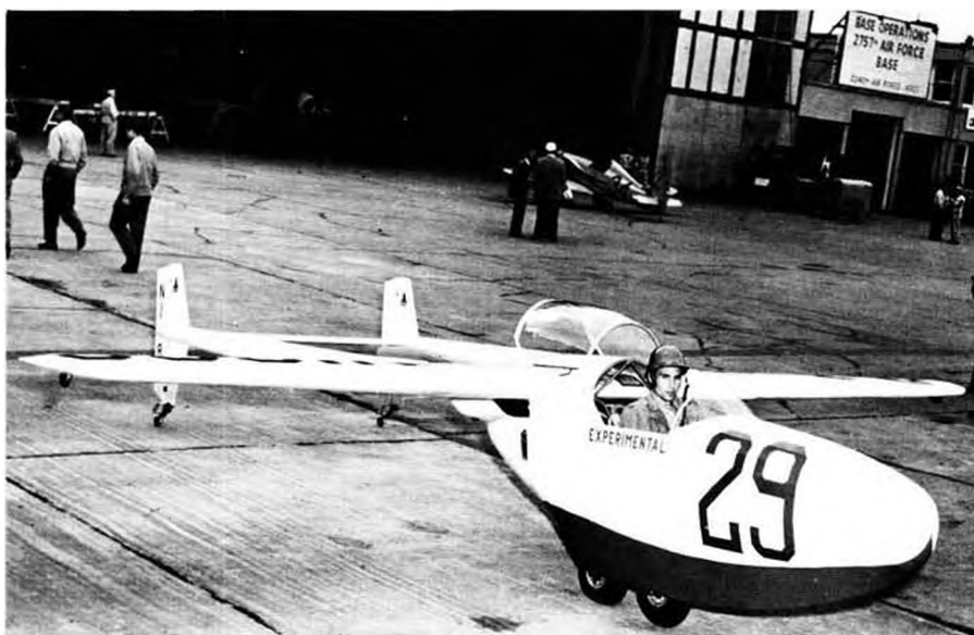
Designed and built by the Lawrence Institute of Technology students, this airplane was later changed to trike gear. Design was never fully explored. Goodyear photo.
