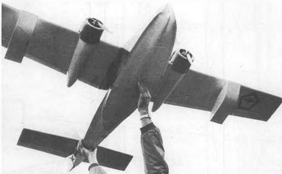
Underside shot discloses the wide hull and spray rails which help prevent water spray from hitting the propellers during takeoff runs. Wide tip floats not as pretty, but very functional.
