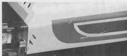
Tear in glass hull caused by collision. Also note propeller "teeth marks."
