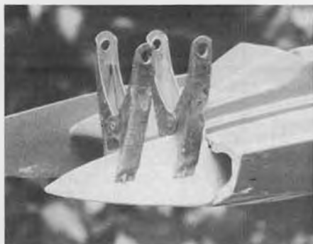
First "sister frame" is spliced inside existing frame, followed by replacement.
