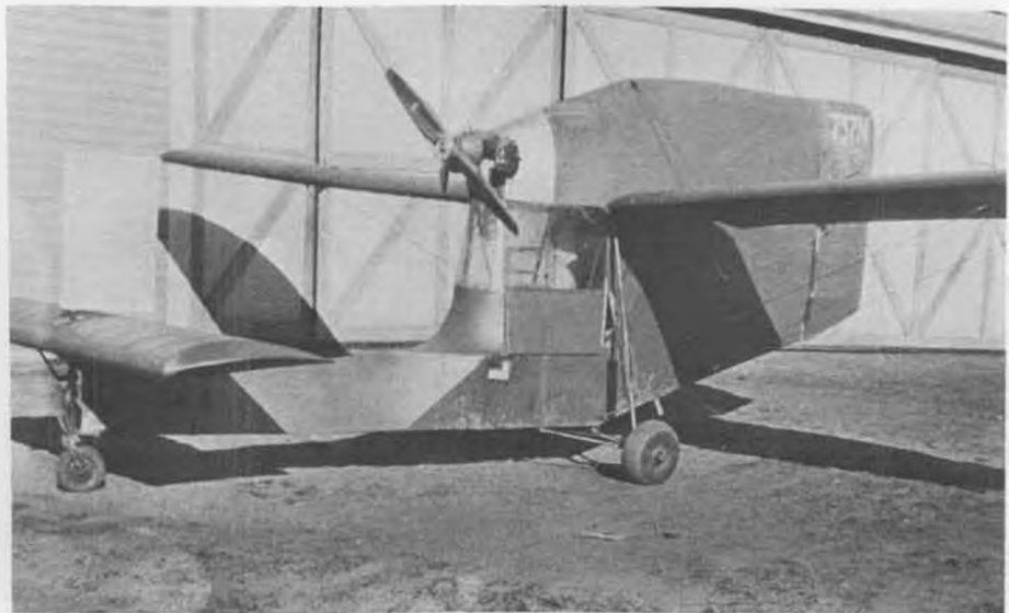
Experimental forward rudder. Normally flat-bottomed Aeronca wings appear to have trailing edge droop. Anyone ready to give it a try?
