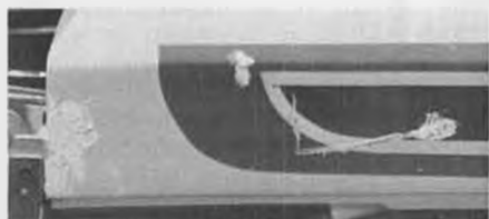
Auto putty used to fill prop marks and repairs to torn area. Sand out and paint.
