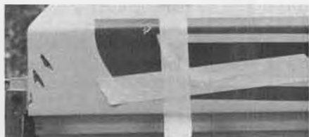
Tape on outside backs up fiberglass resin and cloth applied to inside of tear.
