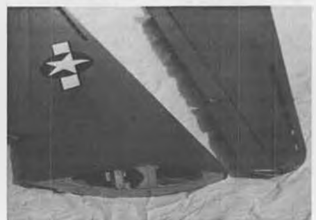
The N9M-A model's wings feature adjustable pitch control surfaces near tips (no servo), elevons, and true-to-scale L.E. slots.
