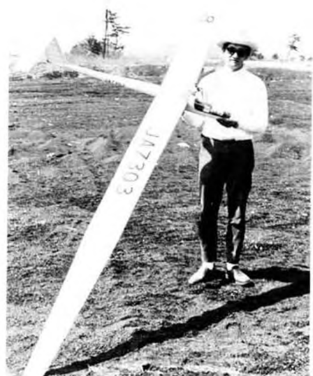
Original design by N. Yamamoto, has flaps, spoilers, rudder, flying stab. OS .10 power.
