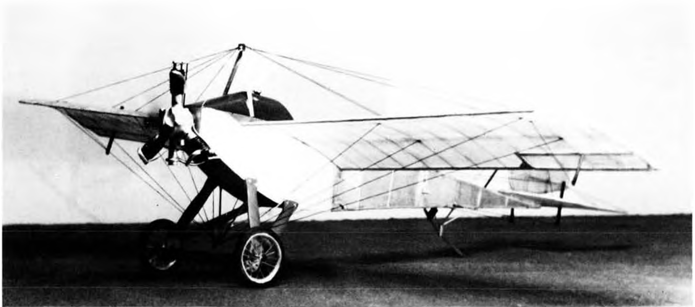
This 1913 E. A. C. Monoplane is by Bill Warner, for rubber or CO 2 power. Span 19-1/2". Design won Senior at 1967 Nats for Mike Mitsch, and CO 2 F/F Scale at the 1970 Flightmasters Annual (This ship). CO 2 engine fits inside dummy motor.
