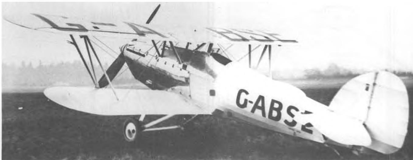
G-ABSE was Hawker PV-1 (Private Venture) Fury, built to test upgraded Kestrel engines, wheel spats, and other mods which led to the Fury II and many export Sales to Spain, Portugal, Yugoslavia, Greece, Persia, and Norway.
