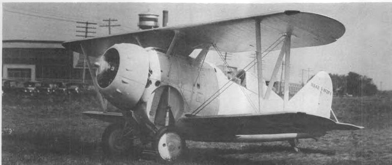
Stubby little bugger, wasn't it? This is the XF2F-1, the first single-seat fighter designed by Grumman and prototype of the F2F-1 in the drawings. First flown on October 18, 1933, the XF2F-1 had a top speed of 231 mph at 7500 feet. Photo courtesy of Ron Clendennen.
