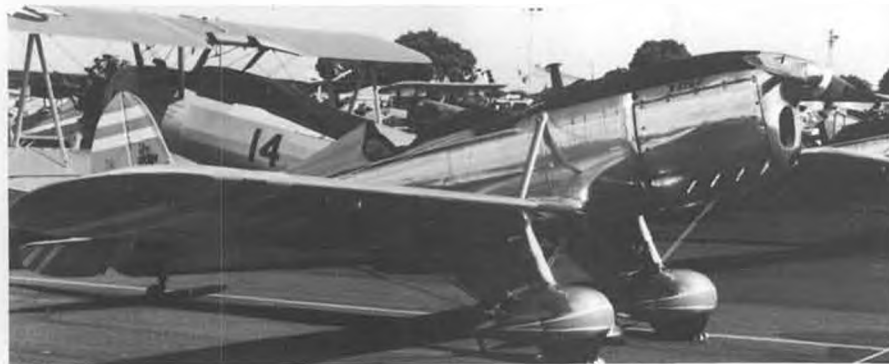
Rearwin Sportster is one of the rarer antiques seen these days. They were built in Kansas from 1935 to 1941 and were usually equipped with LeBlond engines of 70 to 90 hp, with an occasional 90-hp Warner. Fernando says he had a chance to buy one of these planes, in excellent condition, at a Rockford fly-in several years ago for only $2500, and passed it up!
