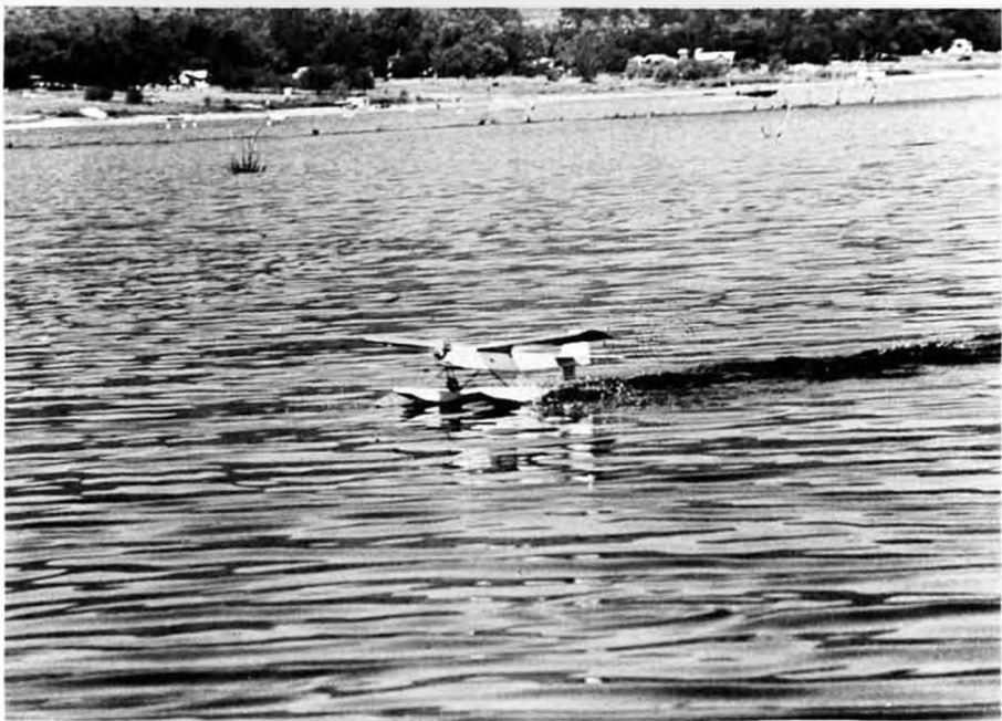
Joe Tschirgi's much-modified H or A-Ray, making a high-speed taxi run to the shore line. As you can see, Joe simply substitutes sled-type floats for the main gear when he decides to go seaplaning.
