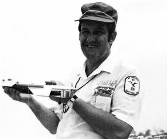
Dick Hall with his very unusual FAI speed plane. Short stroke home-built .15 engine is designed to run at 40,000 rpm!
