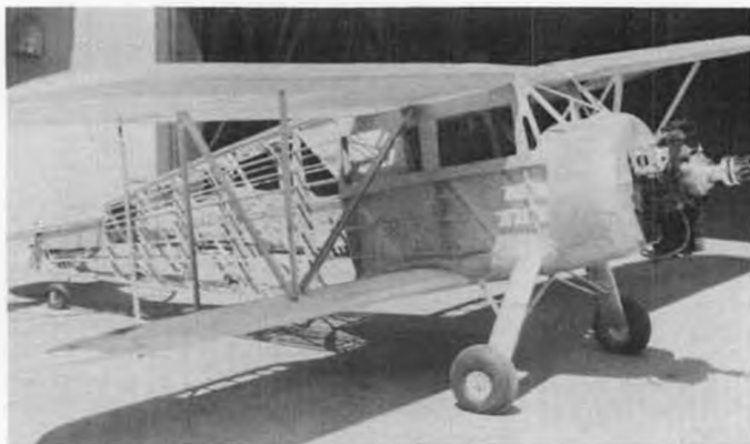
Waco YKS-6 under construction by Dick Igaz, Cupertino, CA. Uses a 3.15 Kawasaki and expected to weigh about 30 pounds.
