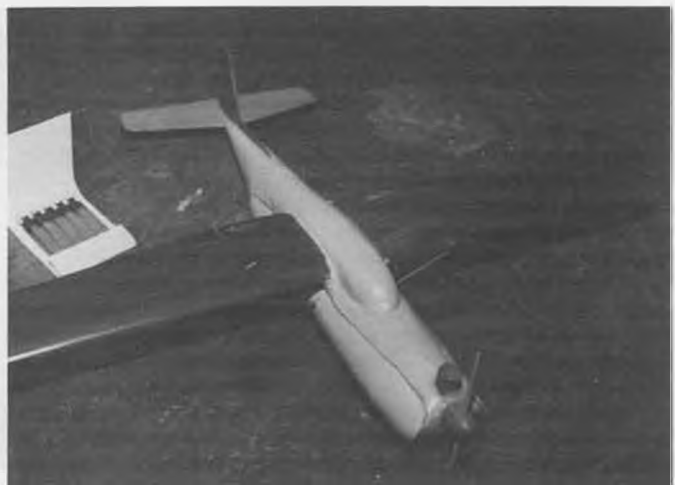
Our author's "Seatract," built back in 1975, was an experiment to determine the feasibility of twin retracting floats. The small scale model shown here, with the floats extended and retracted, was built first to develop the retract mechanism geometry. Discussion in text.
