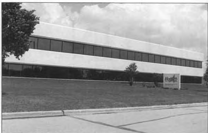
Newest Hobbico office building.
