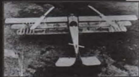
■ ABOVE: Another of Henry Berliner's experiments was this triplane. Here again he used the two big main rotors and also added a small one near the tail. Vanes below the main rotors were for roll and yaw control. ■ LEFT: The first really successful helicopter was the German Focke-Wulf FW-61, first flown in 1936. A radial engine in the nose drove twin counter-rotating rotors mounted on outriggers. A small prop on the front of the engine provided cooling air only, not forward thrust. MB has construction plans for frequent contributor Skip Ruff's RC autogyro version of this same machine: it's plan #4751, $10.50 plus $4 S&H.
