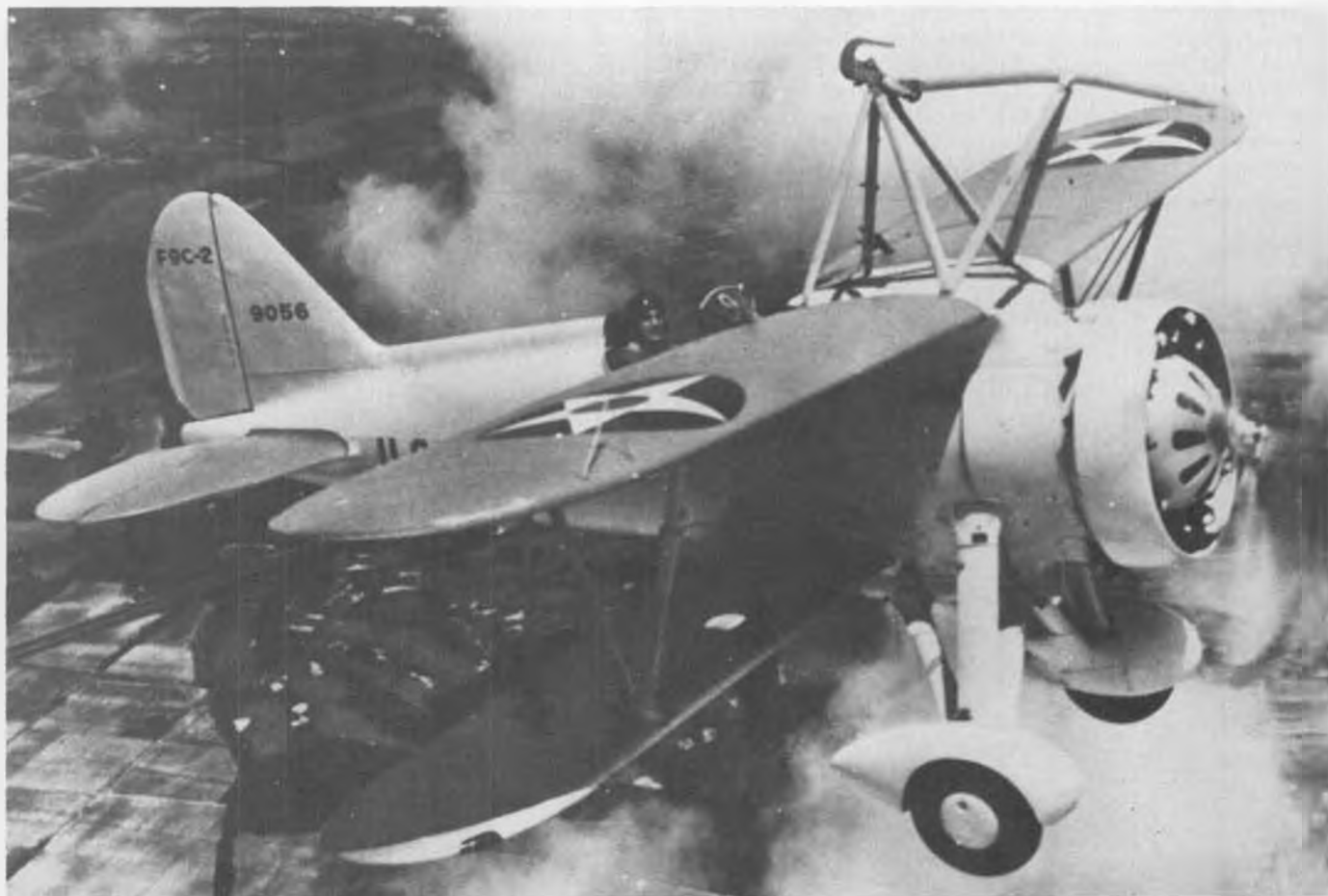
Prior to photo of 9058 above, 9056 in flight photo shows first increase in vertical tail area to overcome turbulence created by hook structure, a 2-7/8" wide strip on trailing edge of rudder.
