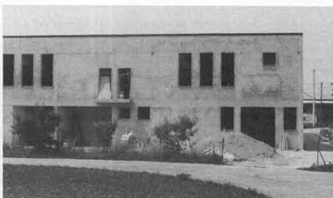
To meet increasing demand for the Rossi engines, an additional manufacturing building is under construction.
