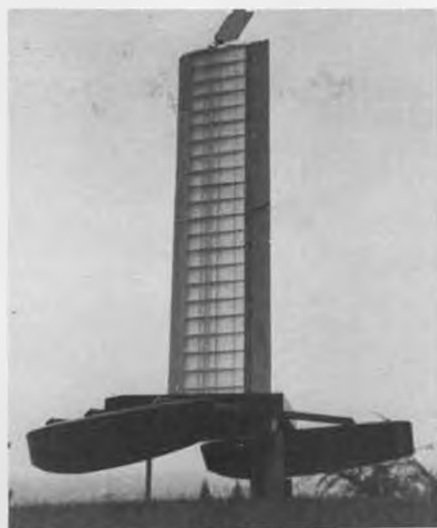
CD Min's predecessor was this catamaran, called "CL Max." Wing construction on both boats is balsa with doped silk covering.
