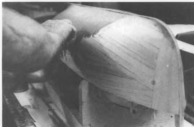
After saturating interior of planking with epoxy, the exterior is rough sanded and then a coat of Sig Epoxilite is added.
