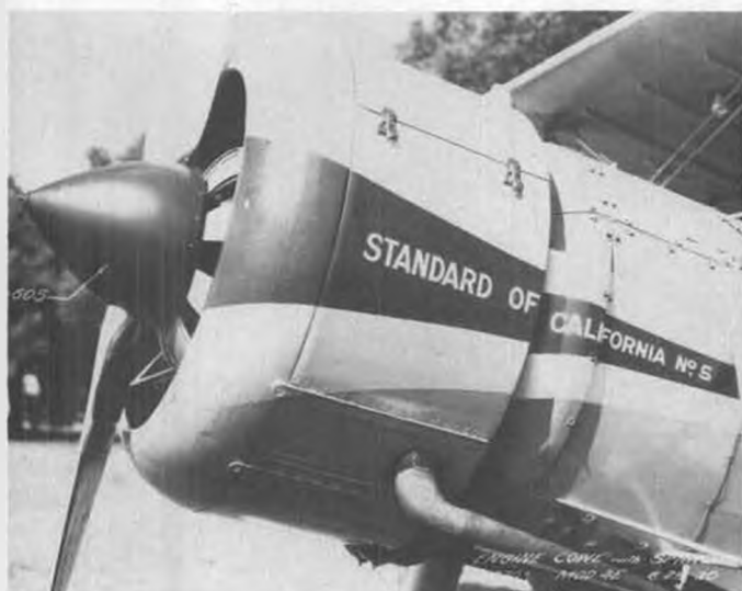
Handbook photo of Stanavo 4E shows excellent detail of suitcase cowl fasteners and numerous twist fasteners.
