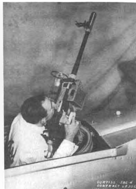
Tail gunner had a .30 caliber Browning on a horseshoe rack. Right and left hand and shoulder grips were provided. Nat'l Archives photo.
