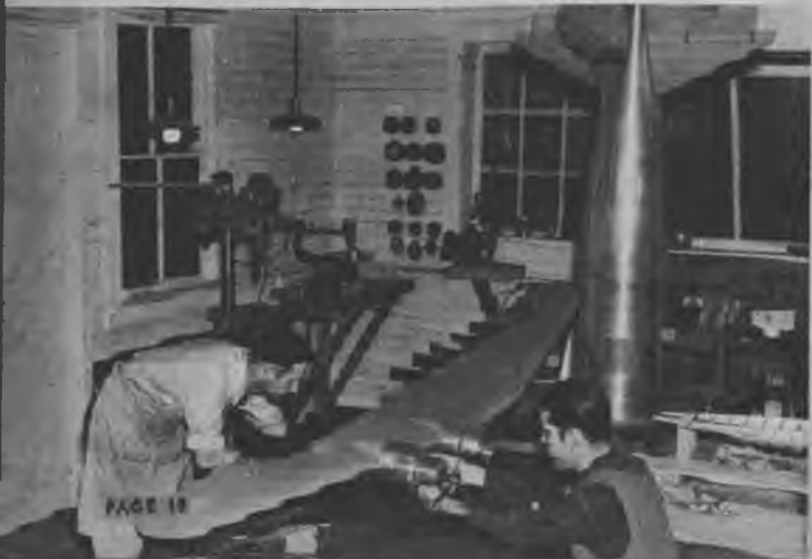
What model builders dream of. This complete shop at Boeing turned out $10,000 model of the Stratoliner, among others. Body was of spun aluminum made in sections.
