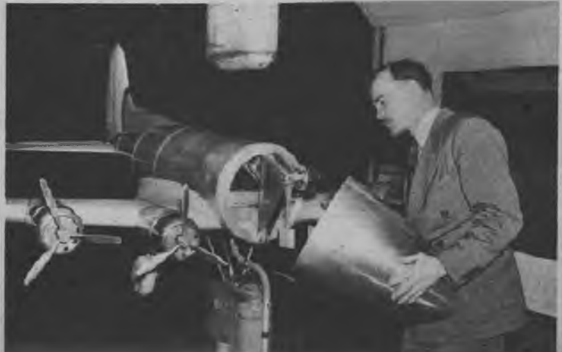
Test pilot Eddie Allen investigates automatic control system of baby Stratoliner. Miniature electric motors drive propellers to simulate flying.
