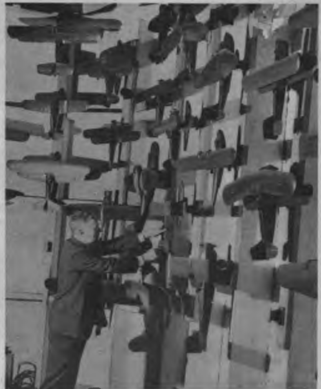
Wind-tunnel models require extreme accuracy and many hours of work. Engineers depend upon findings of tests for predicting full-scale results.
