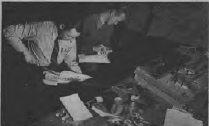
NAGA modelers attribute their skill to model-plane building: construct wind-tunnel models from wood to tolerances normally required only in metal work.
