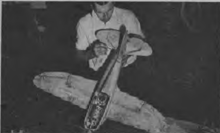
Andy Yeryzer with an electrically driven F-35. Model is used in free flight tunnel. Electromagnets activated by impulses transmitted by wire work controls.
