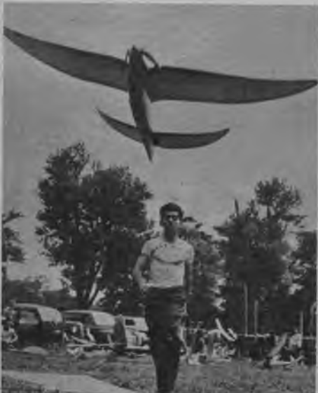
● Here is clean design—note the elliptical wing and stabilizer dihedral, also the folding propeller.
