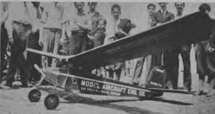
● The 1935 KG is one of the really famous planes. Its record of 64 minutes still stands. It features a parasol wing and wingspan of 10'; weighs 7 1/2 lbs.
