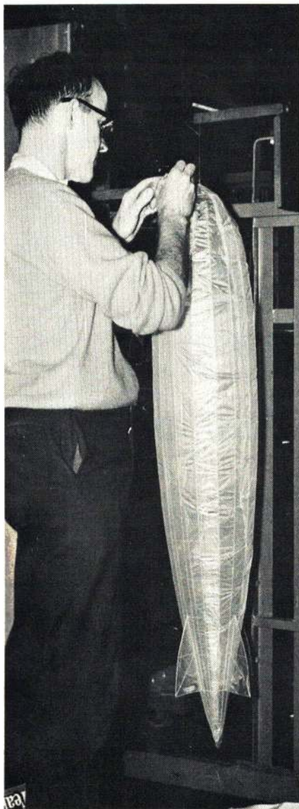
Above: That hull is a form of art. A sneeze could destroy it! Right: The monster climbs only from propeller power. Flight attitude is adjusted by the weight at the end of those strings. Below: One of Bill's most unorthodox indoor jobs, and clearly the largest, is the dirigible. It is rubber-powered. Left: To fly, it needs a bit of gas. It is not pressurized at all and is adjusted for slight negative bouyancy.
