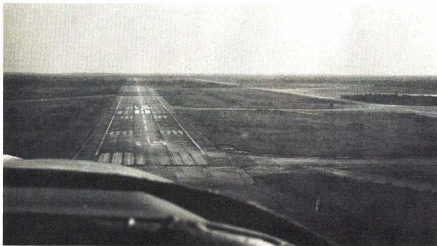
View of Chennault Airport from a lightplane. Note that the runway directly ahead goes practically to infinity—12,000 feet long and 200 feet wide! It's big by any standard.
