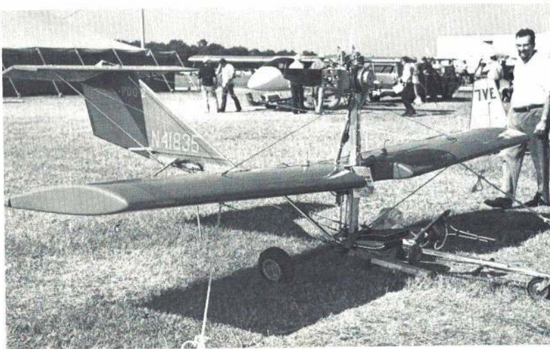
Right: Wayne prepares to take off with an engine that will cruise at 70 mph. Below: Wayne Ison's PDQ-2 is a study in simplicity. You can even use a discarded engine for power. Below right: Wayne discusses the engine—a snowmobile engine—with the author.
