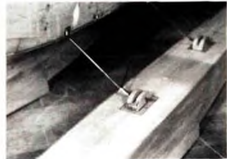
Close-up of strut blocks, spreader bars yet to be added.
