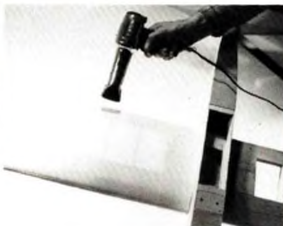
In a continuous sweeping motion, use heat gun for final shrinking.
