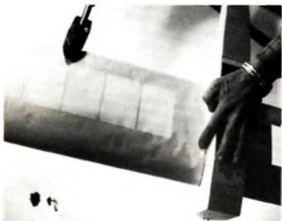
Lay material in place and tack down at intervals before sealing completely.
