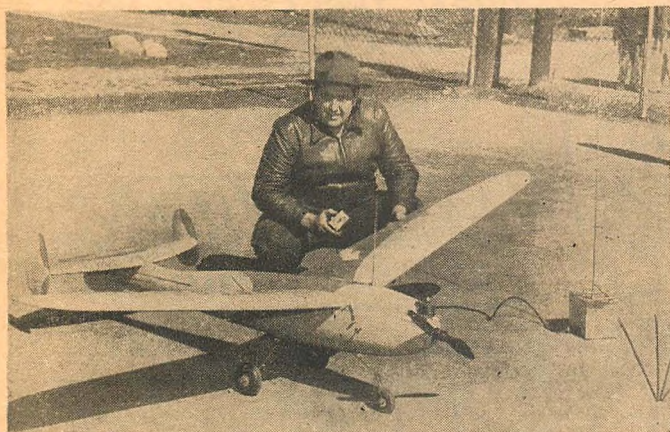
No. 9 R. B. Spencer's Custom Cavalier R. C. plane using audio tone control
