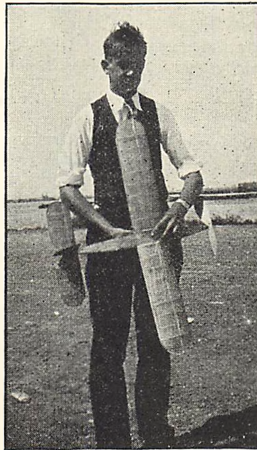
Gordon Light of Lebanon, Pa., carefully designed his propeller for the record-breaking plane he is holding, by means of the formulas and data given in these articles. His ship flew officially for 25 minutes and 53 seconds, covering a distance of eight miles, and establishing a world record
